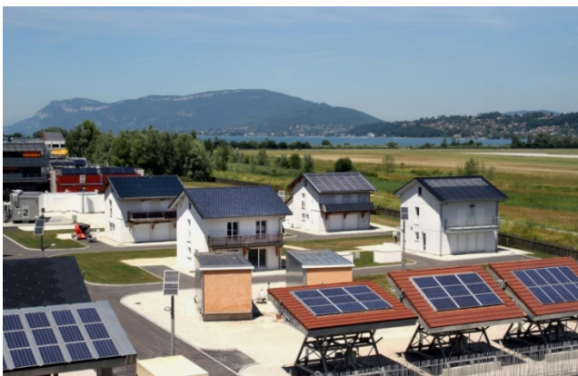
Experimental platform located at the French National Institute of Solar Energy (INES) near Chambéry / France. The experimental platform is used for testing novel materials and systems, e.g. by the EU funded HOMESKIN project ( https://homeskin.net/ ) in their development of thinner insulation systems and by other EU-funded projects Source: INES Platform
