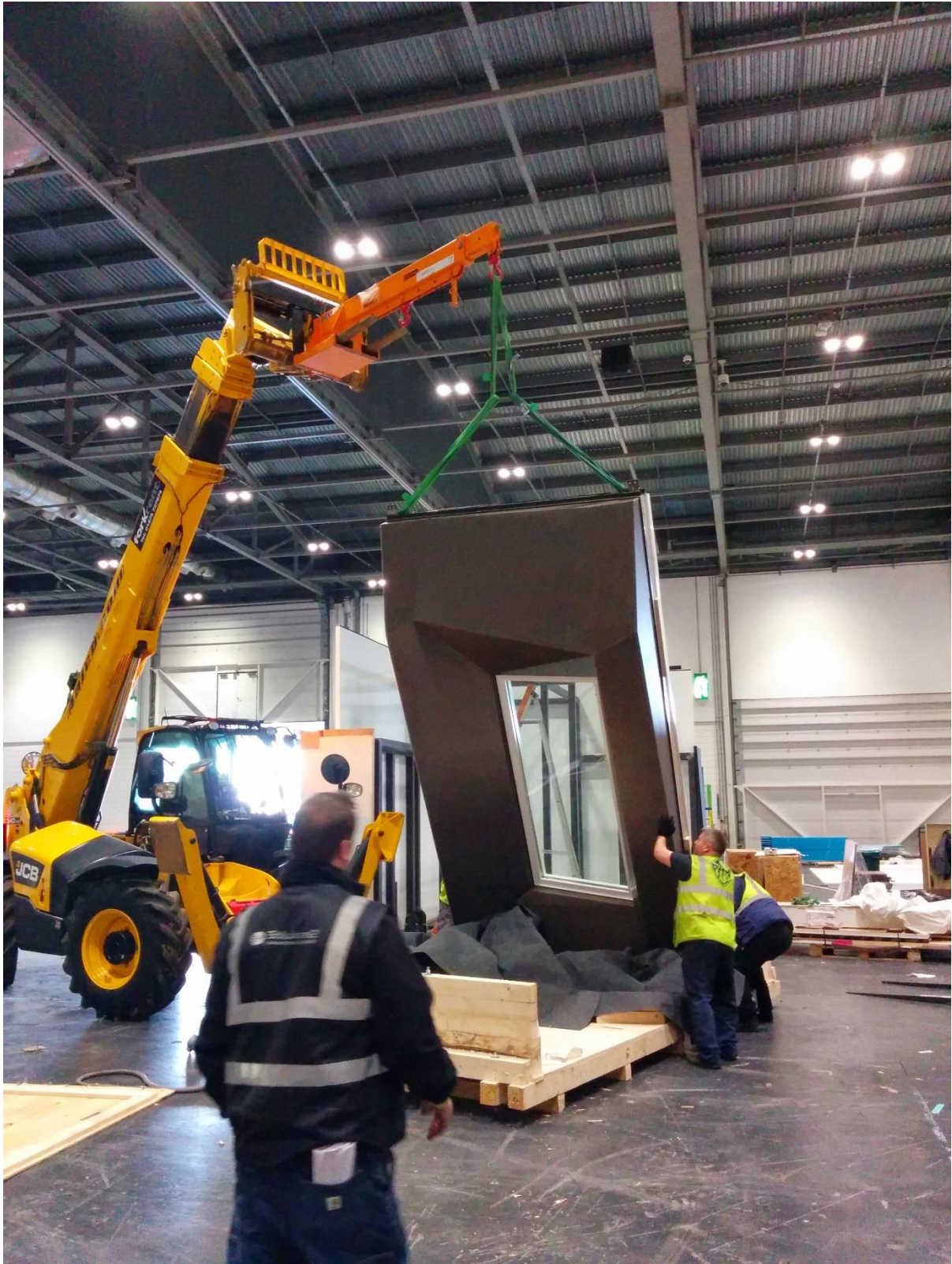
Figure 3. Erection of the EWP.
