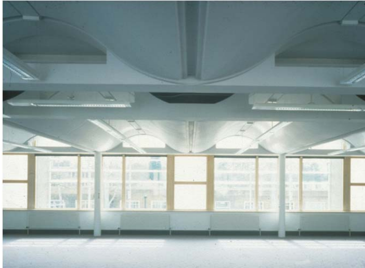
Exposed thermal mass of concrete structure in an office building
