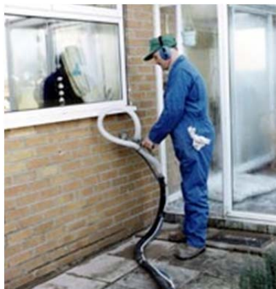
Injecting a cavity wall with full fill insulation
