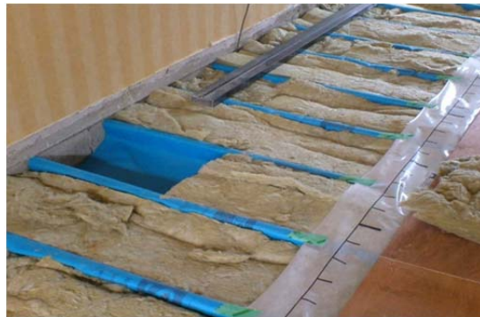
Retrofitting an airtightness membrane and insulation to a timber floor.
