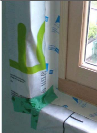
Retrofit airtightness detail at window / wall junction.
