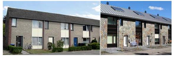
Figure 7 Roosendaal before (left) and after (right) renovation (Photo: Chiel Boonstra)
