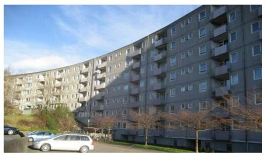
Figure 3: A typical house with prefabricated elements and visible joints from the post-war era.
