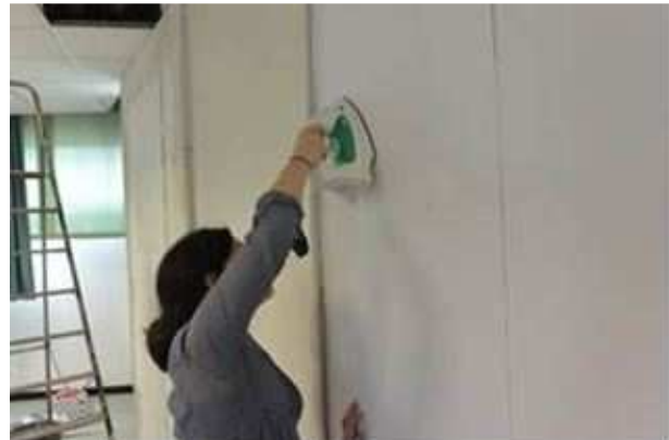
4 - Encapsulating textile glued to the aerogel.
