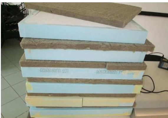
1 - Storage of perlite boards with frame protection before installation.
