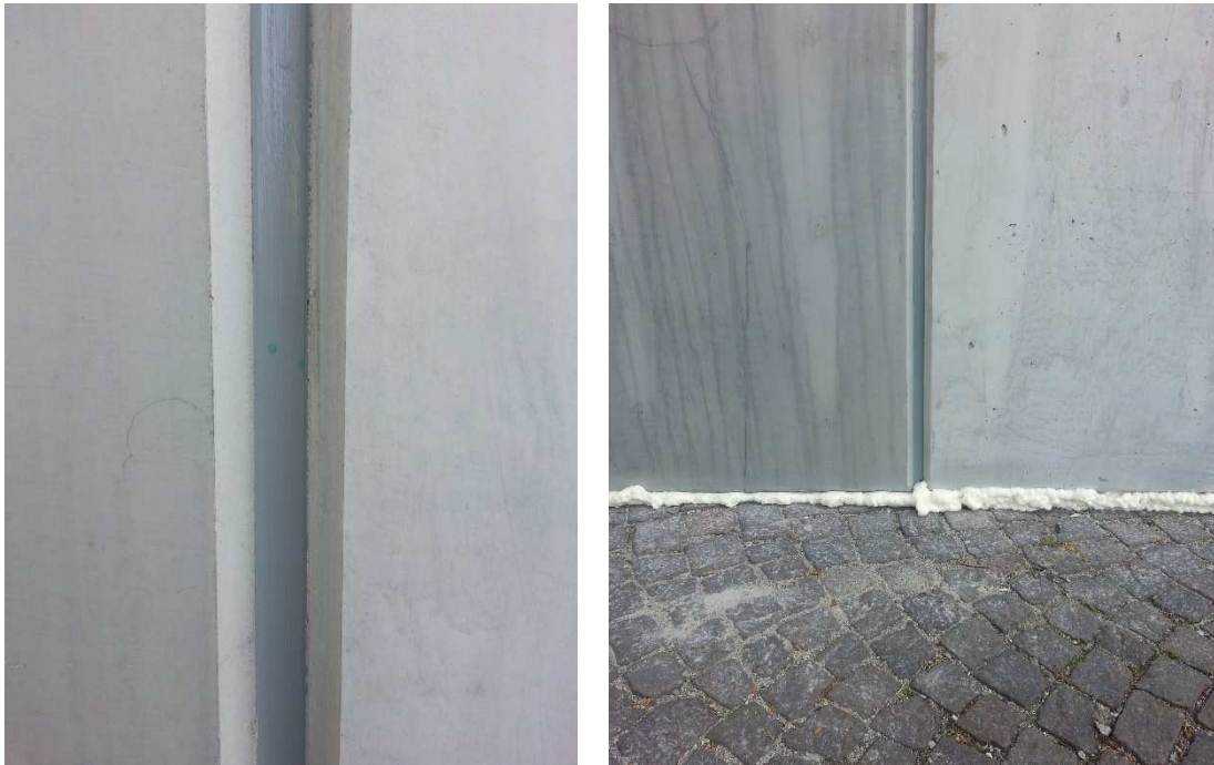
Figure 1 – The grey silicon sealant between the panels and the polyurethane foam
