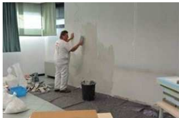
2 - Implementation of the grounding layer for the perlite insulation board installation.
