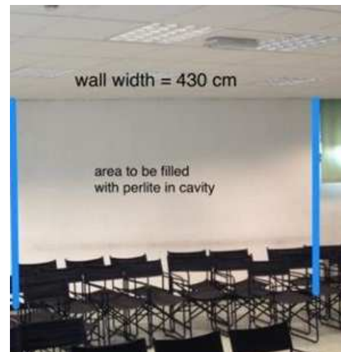
Figure 5: Inner view of the room before retrofitting through perlite injection
