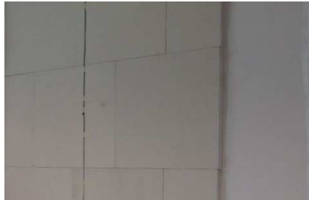
4 – Fix all the panels on the wall, before applying mesh, protective corners, filler and base coat.
