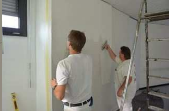
6 – Application of a resin overcoat – finishing layer.
