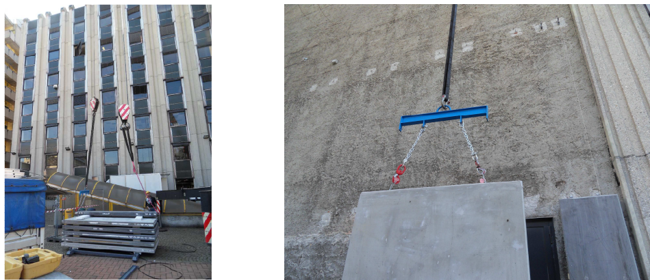
Figure 19: Panels storage and handling
