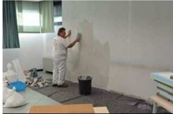
2 - Implementation of the grounding layer for the permeable insulating wallpaper installation.
