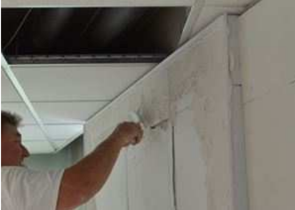
5 – Application of mesh, corner protection, filler and base coat.
