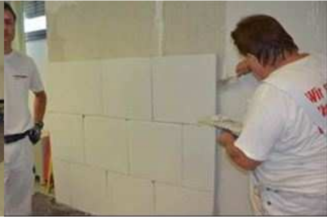
4 – Application of the further lines to cover the wall.
