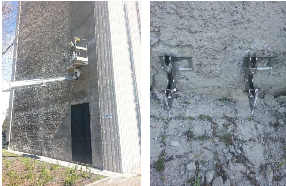
Figure 23: Pictures of the installation phase
