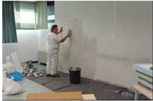
2 - Implementation of the grounding layer for the flat laminated panels installation.
