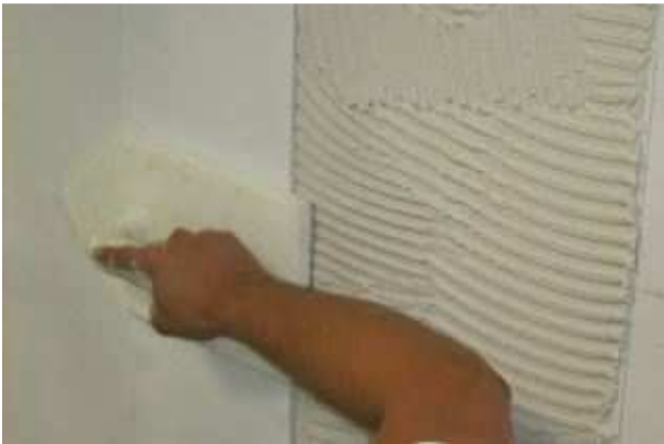
3 - Application of the wall-paper on the grounding layer.
