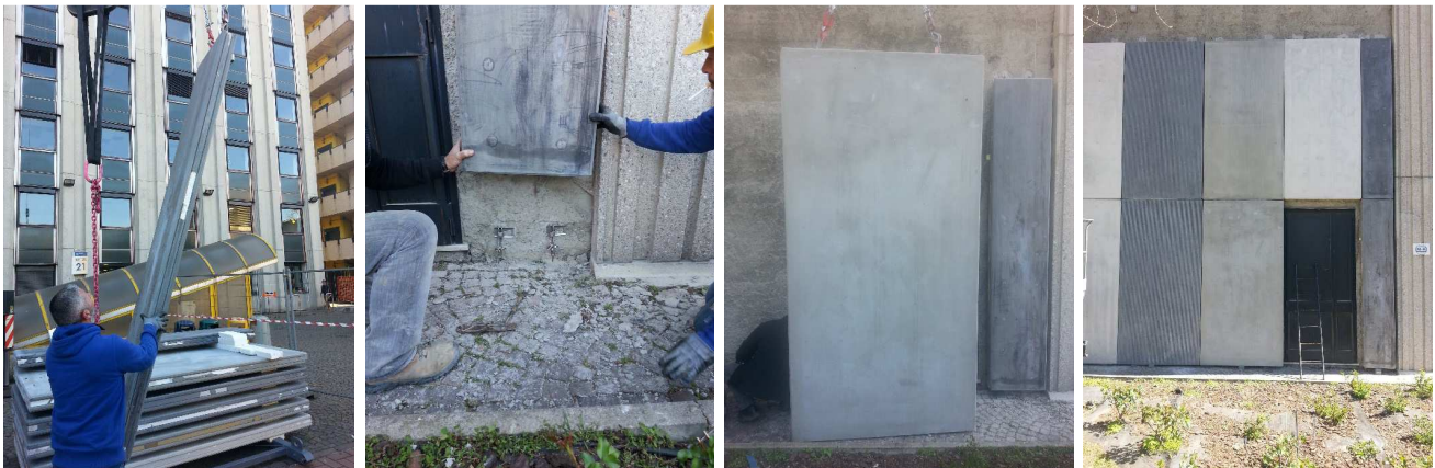
Figure 24: Some pictures of the installation process
