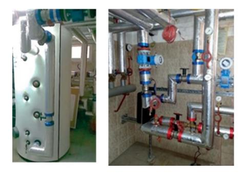
Photo 2. Boiler and its equipment installed room after modernization
