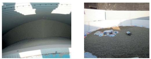
*Photos 8 and 9. Detail of the insulation of the space between both metallic tanks and the bottom part.*
