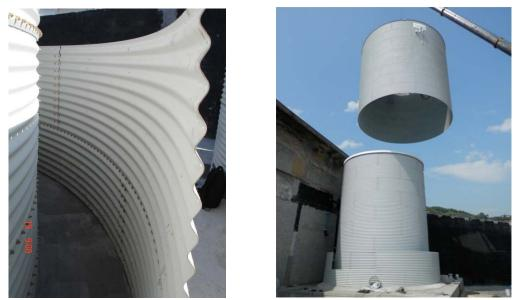
Photos 6 and 7. Detail of the corrugated galvanized sheet bolted steel and the double tank system
