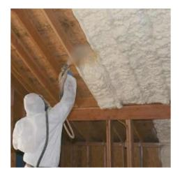
Figure 6 : Foam thermal insulation technology
