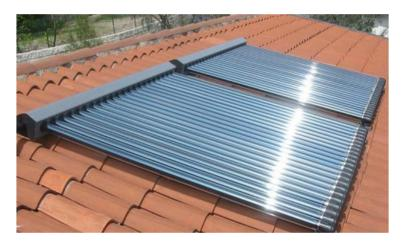
Figure 39 : Vacuum tube solar water collector
